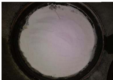
Manhole insert at installation
