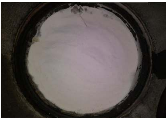
MH insert at install
