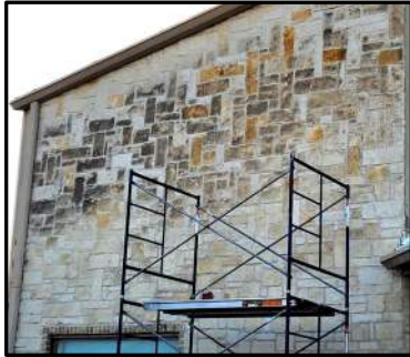
Figure 2: Left (N.W.) side of Texas limestone church stained by mold and pollutants prepared for deep cleaning.
